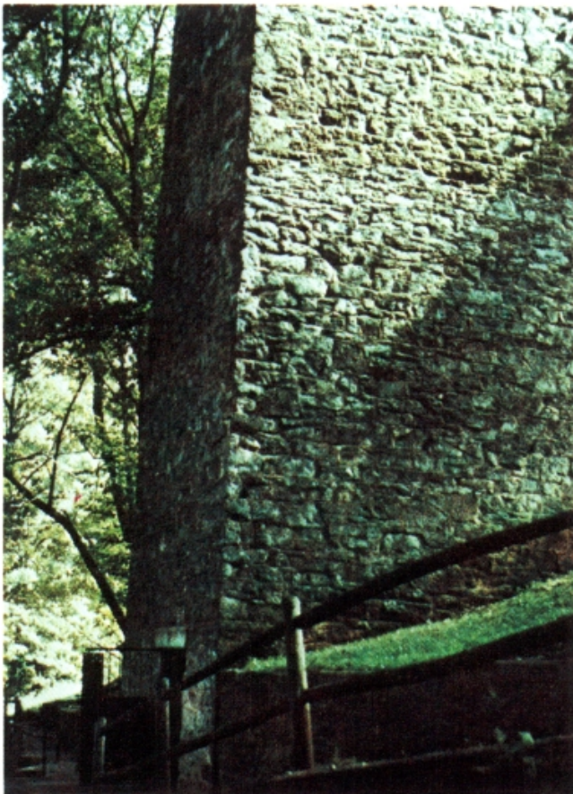
West Side and Entrance at Rear (North) Wall
