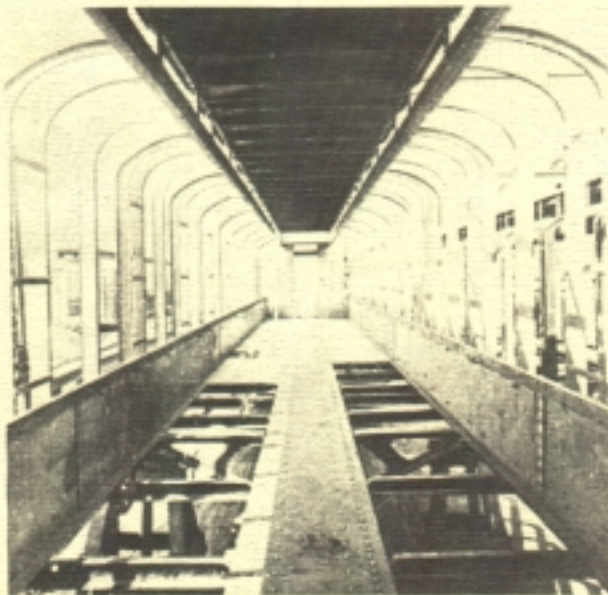
The car structure combined steel castings with rolled steel shapes and plate. The heavy center sill is the primary structural member. (Pullman Neg. 12484)
