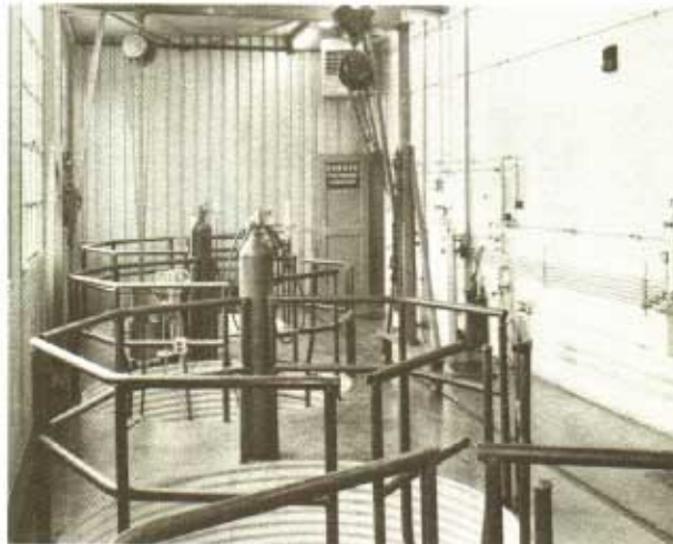
FIGURE 5. View of Battelle's new gas-pressure bonding pit bay in 1958.
